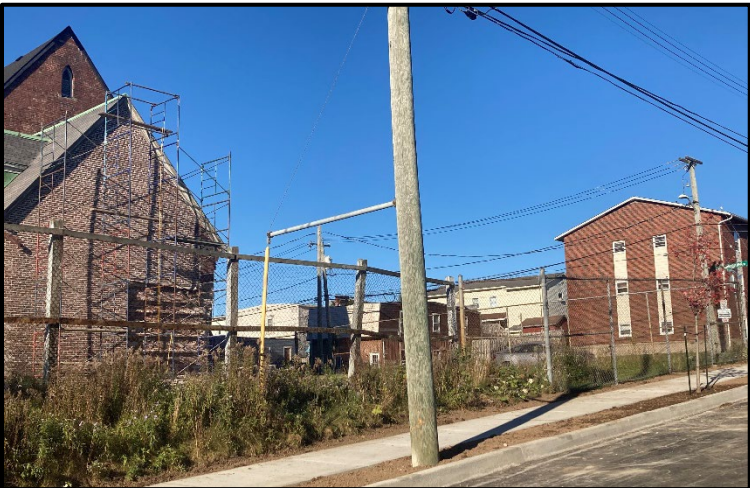
Photo: Adjacent properties to the east of 54 Broad Street
