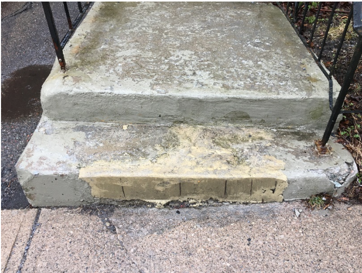
View of prior repair work. West landing.
