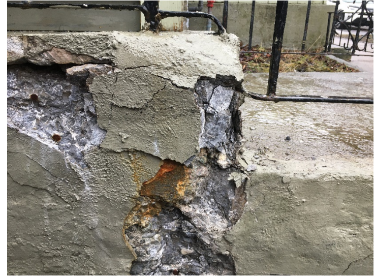
View of water-infiltrated spalling concrete. West landing.
