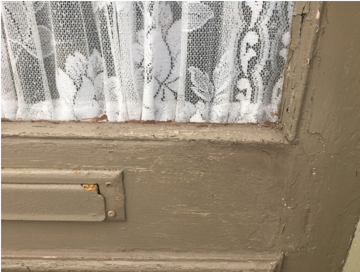
View of deteriorated filler around glazed panel on South-facing door.
