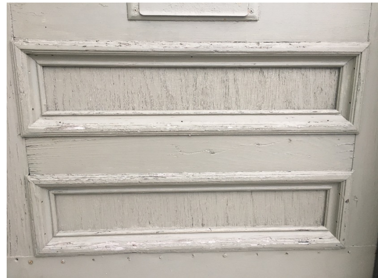
View of deteriorated plywood panels on West-facing door.
