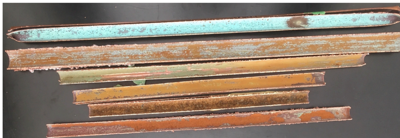
Figure 1. Sections of copper pipe cut longitudinally for scale analysis.
