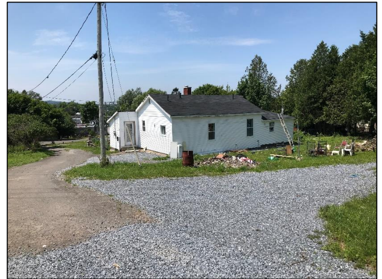
View of existing dwelling on site.
