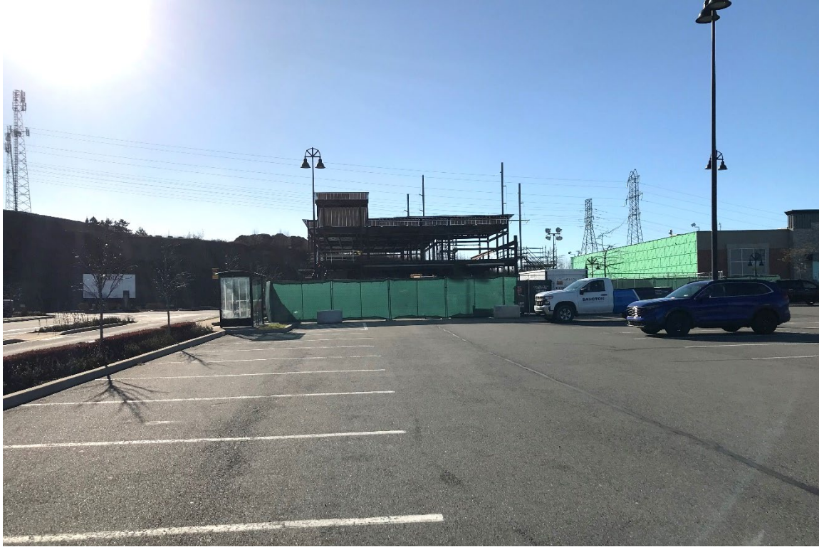
Building Under Construction – 24-32 East Point Way (PID 55230445)
