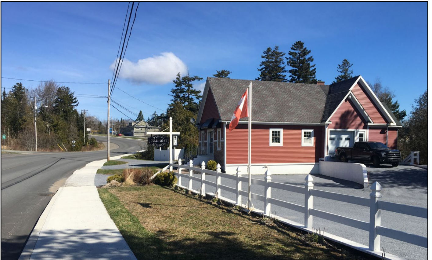
Subject Site looking North up Westfield Road
