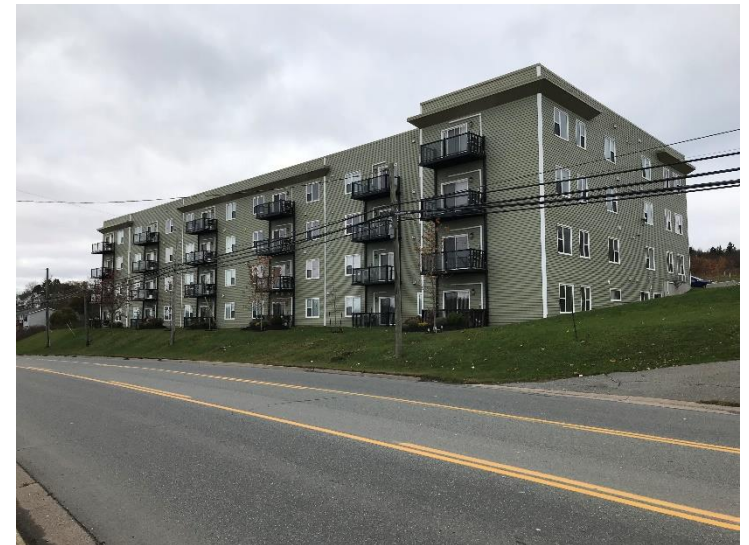
Existing building topology on Loch Lomond Road.
