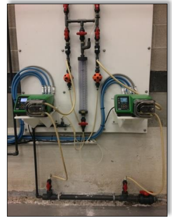
Figure : Temporary Orthophosphate Dosing System - Spruce Lake WTP
