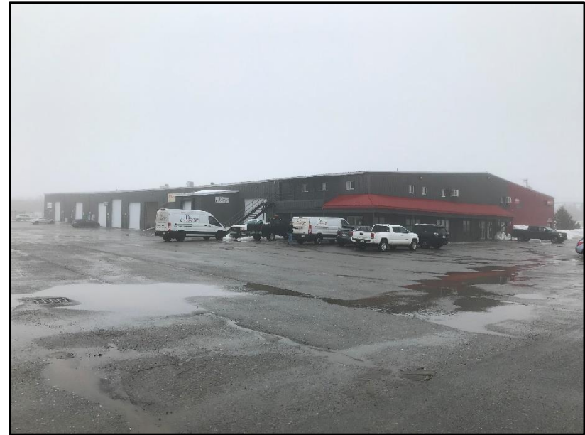
View of existing building.
