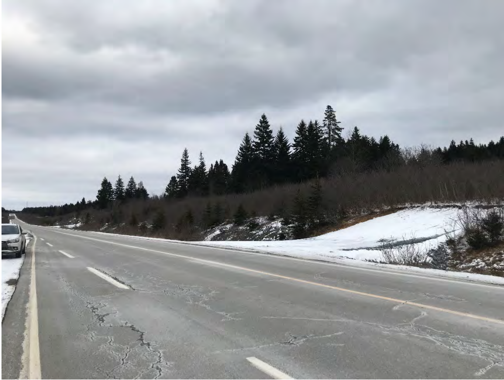
Quarry access (left) and Subject Site Access (right)
