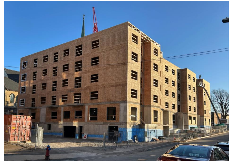
Steepleview Development (under construction) 35 Cliff Street 56 Units / 28 Affordable Units + Daycare
