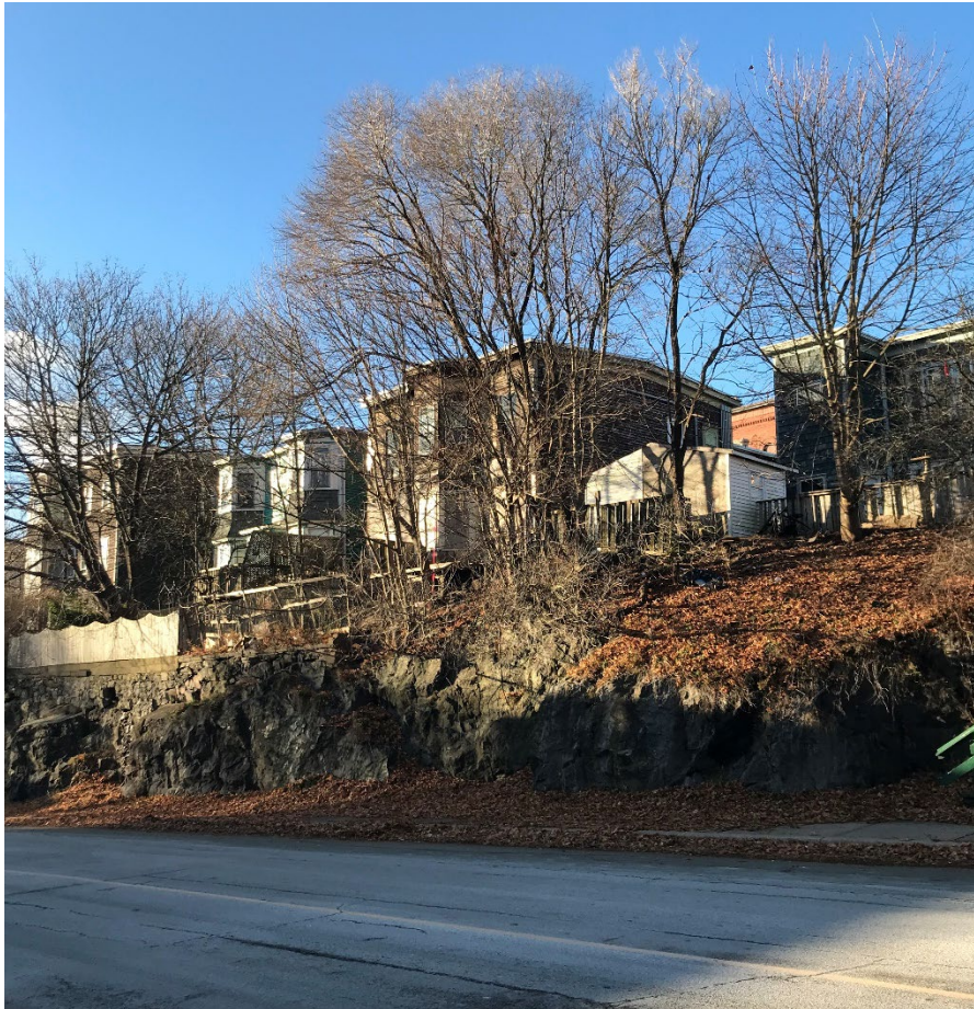
9 Waring Street - View from Main Street
