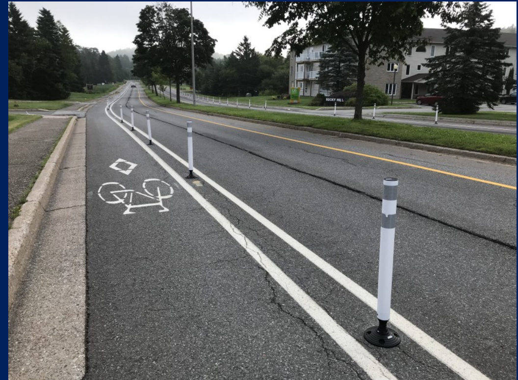
Option would be like University Avenue, pictured here. 1 vehicle lane and 1 bike lane on each side of road.
